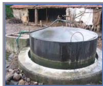
Rural Energy Systems
